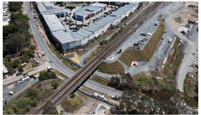
Aerial image of works near the rail bridge on Goldmine Road: October 2026
